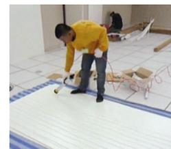
7. Take a start/end U-profile and partially fill it with Food Safe Sealant white. Push the profile onto the bottom end of the CleanSheet.
