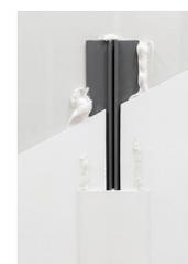
*With HygiSeal:* Stick the PolySto CleanSheet on the wall and press lightly. Adjust the position of the plate if necessary. Use a laser to make sure it's perfectly vertical aligned. Then press well.
