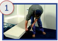
• Hammer the anchorages in the pre-drilled holes.
