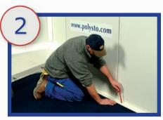
Measure and sign off where you have to drill holes in the floor by using a mould. (available as a 'PolySto' accessory)
